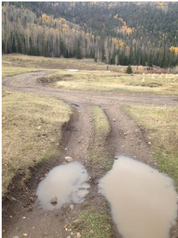
Figure 2. FSR 390 stream crossing that will be hardened with gravel (a) and the stretch of road approaching it (b).
